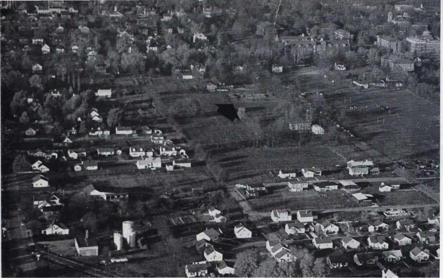
LOOKING DOWN on Oxford, Ohio, from the South the excavation for the new Central Office Building is in the center of the picture as indicated by the black arrow. In the upper left of the photo is the business district of Oxford, with Miami University to the right of the Central Office Building. In the
