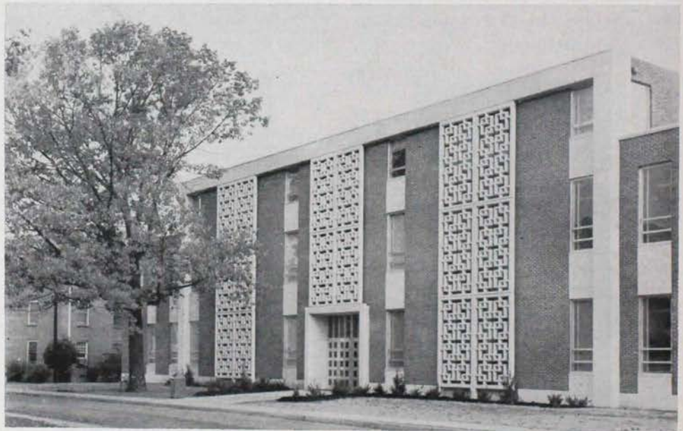
THIS NEW SCHOOL of Commerce and Business Administration Building has just been occupied at the University of Mississippi in Oxford, Mississippi.
