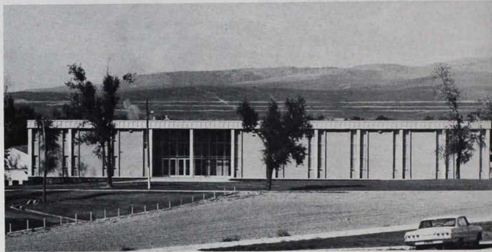
THIS MODERN two story structure is the Leslie J. Savage Library at Western State College of Colorado in Gunnison.
