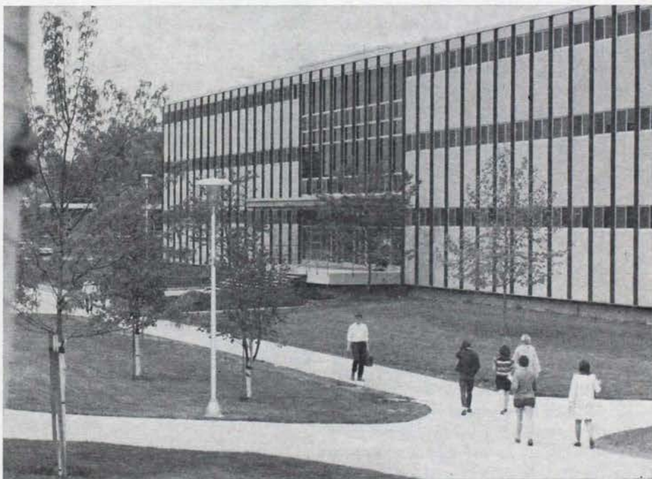
THIS MODERN BUILDING is Upham Hall on the campus of Wisconsin State University at Whitewater where science classes are held.
