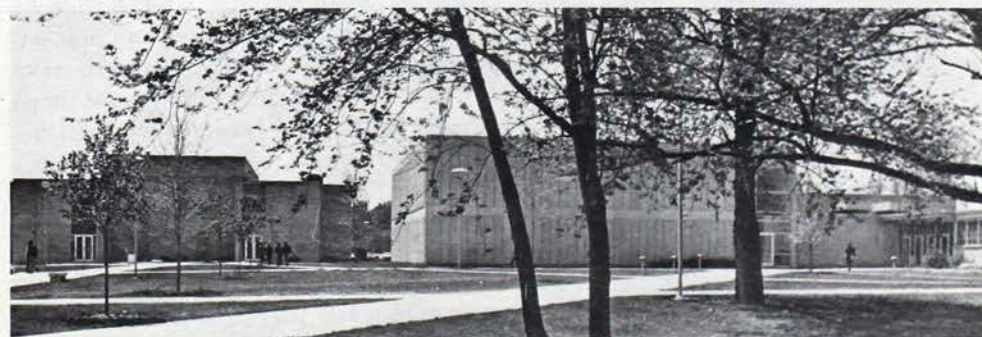
IN THIS SCENE on the campus of Indiana University Northwest at Gary can be seen the Academic Building, Library and Gary Main Building. Indiana University Northwest is the home of Delta Sigma Pi's Theta Psi Chapter.
