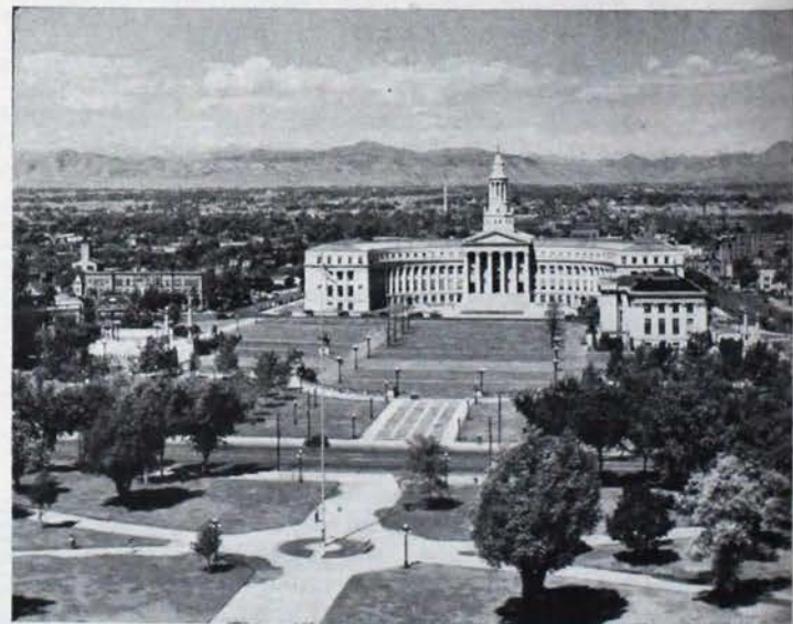
THE CITY AND COUNTY BUILDING of Denver is located in beautiful Civic Center very close to the Cosmopolitan Hotel, the headquarters for the 19th Grand Chapter Congress.
