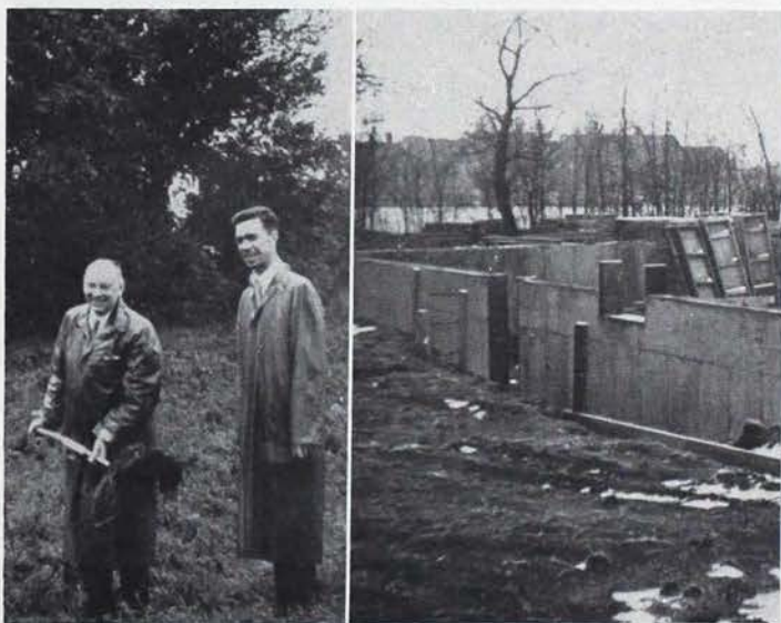
GRAND PRESIDENT J. HARRY FELTHAM officially breaks ground for the new Central Office Building at Oxford, Ohio, while Homer T. Brewer of the Executive Committee looks on in pouring rain. RIGHT PHOTO: Foundation of the new Central Office Building and the construction completed as of December 1.
