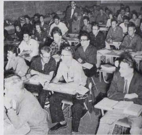
A TYPICAL CLASSROOM in the new College of Business Administration Building at Nevada features a variety of equipment and facilities.
