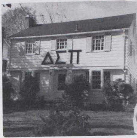
A NEW COAT of paint and large black Greek letters have added much to the Beta Pi Chapter house at Kent State University in Kent, Ohio.
