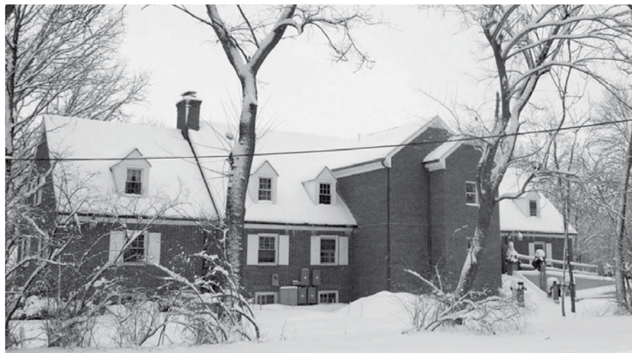
Looking southwest, the new elevator/restroom addition stands out. The new wheelchair ramp is at the far right.
