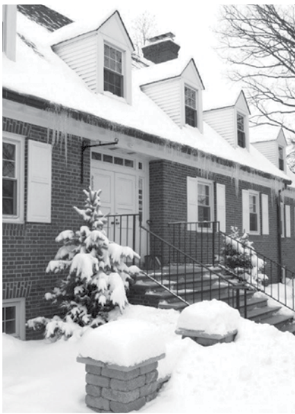
Pretty, yet problematic, record snow and ice added to renovation delays.
